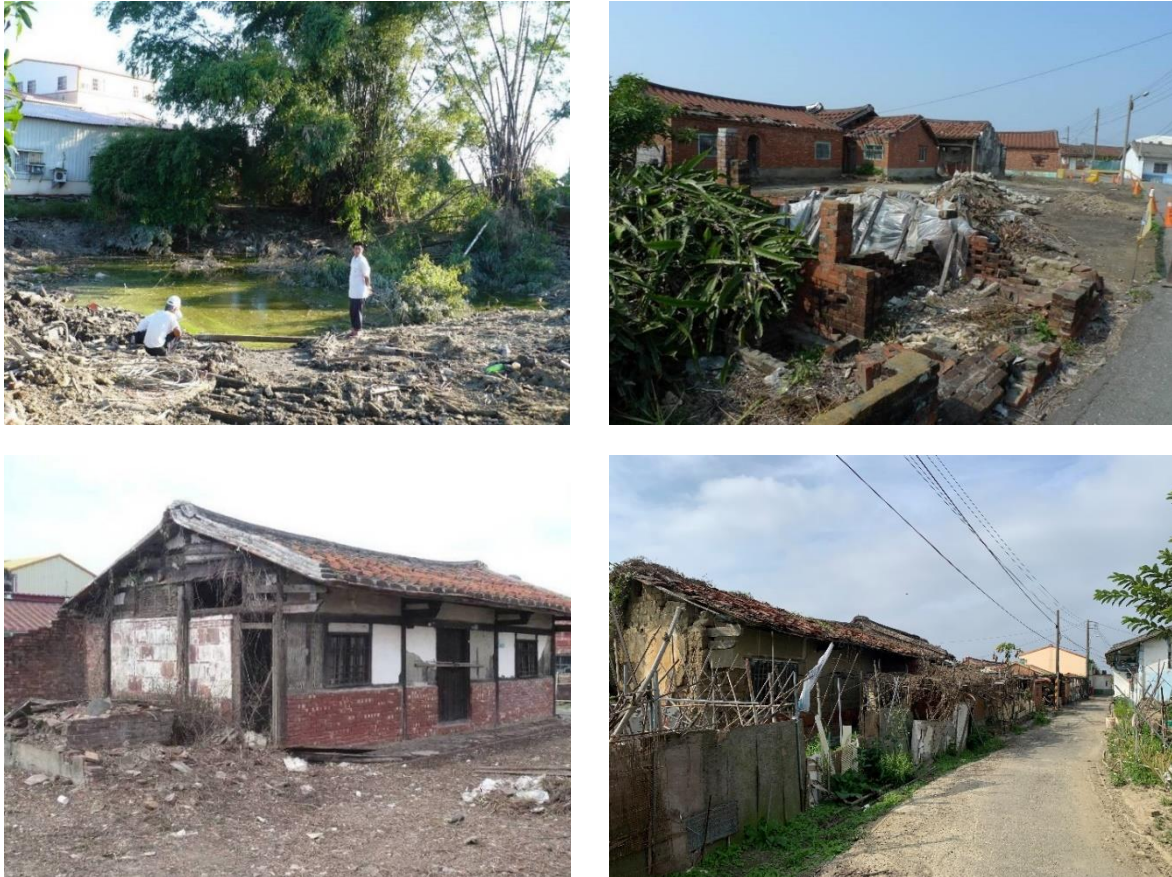
Figure 14: Polluted farm ponds and dilapidated places in Picheng 5
